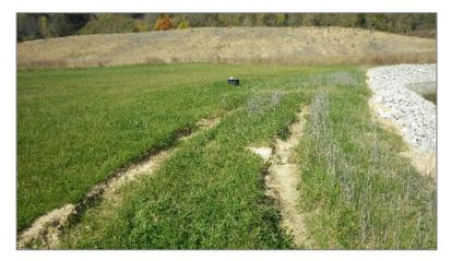
Photo 30, Point 32 Northeast Leachate Pond – Tire rutting near its perimeter.
