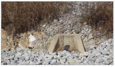
Photo 33, Point 35 Northeast Sedimentation Basin – Headwall to truck washing station.
