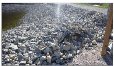
Photo 5, Point 5 Southwest Leachate Pond – Geotextile fabric exposed in riprap protection.
