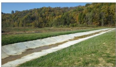
Photo 2, Point 2 Lined stormwater channel adjacent to Southwest Sediment Basin.
